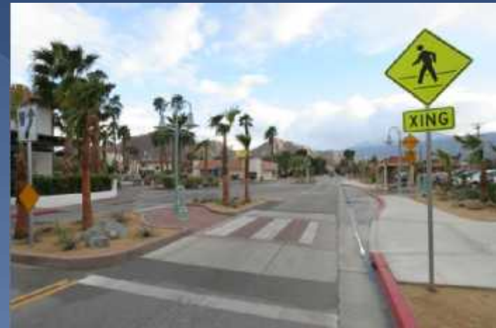
A pedestrian crossing that provides convenient access to a bus stop. Photo by Dan Burden
